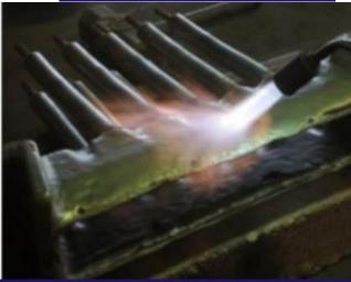
The wear of Core Brick Bridges is minimised and repaired by using an Oxygen Acetylene Hard Facing powder spratorch to apply Tungsten carbide in a 60 HRc Nickel, Chrome Boron matrix.
